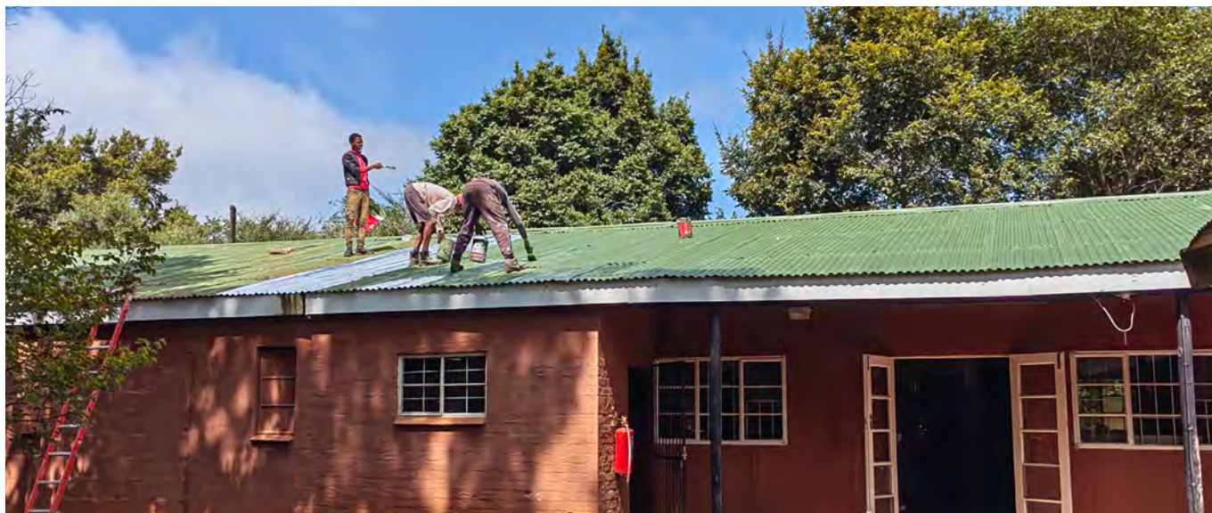
Renovations to the reserve's Education Centre and main office building
